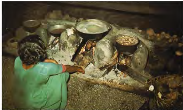
A traditional Maldivian kitchen is located in a separate building to keep a possible fire hazard from spreading to the main house. The hearth is made up of large stones that are periodically covered with a mixture of ashes and saltwater to reduce cracking. (Photo: B. Koehlin)
