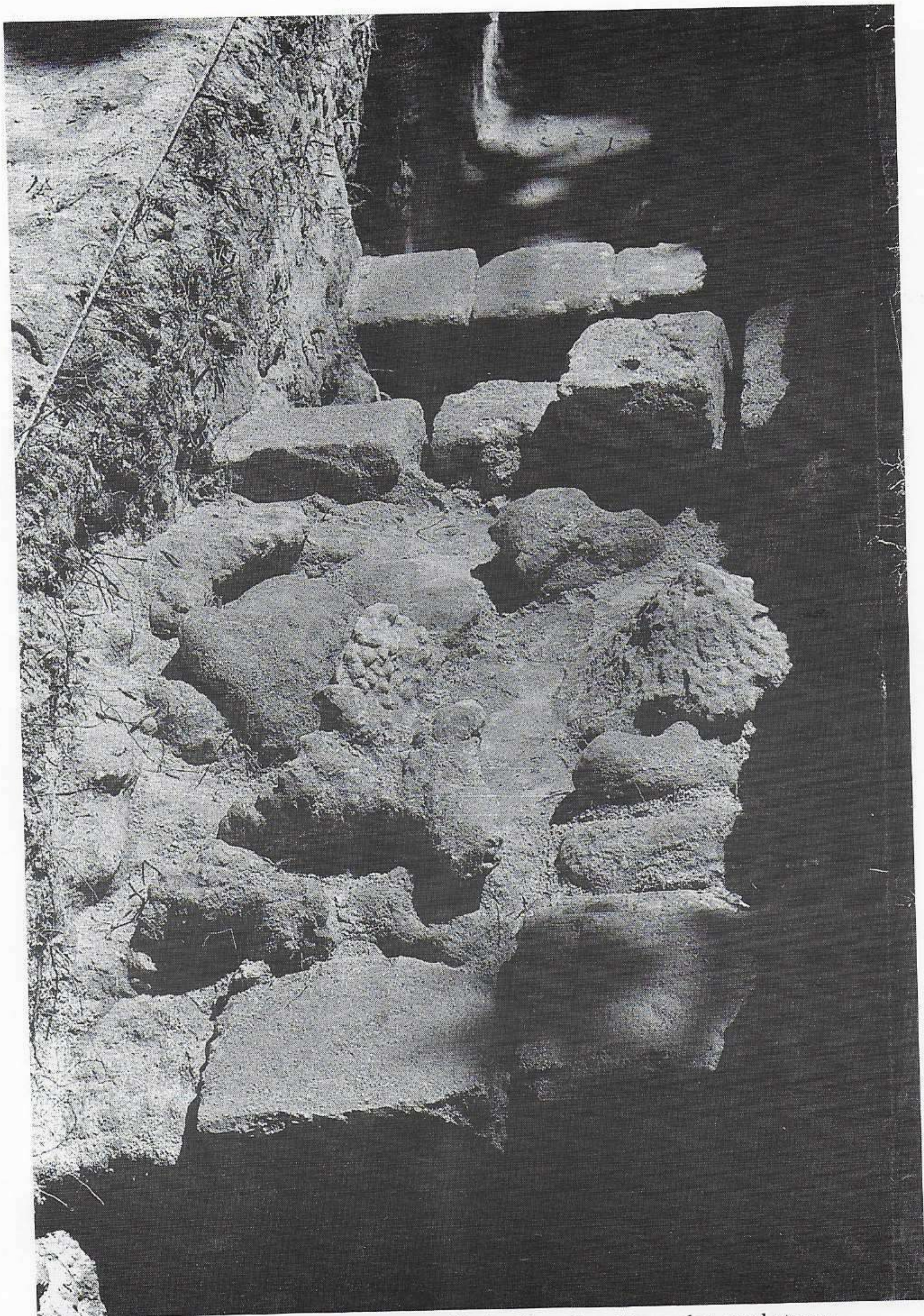
Fig. 2. Big wall made of stone blocks and filled with soil and irregular coral stones.
