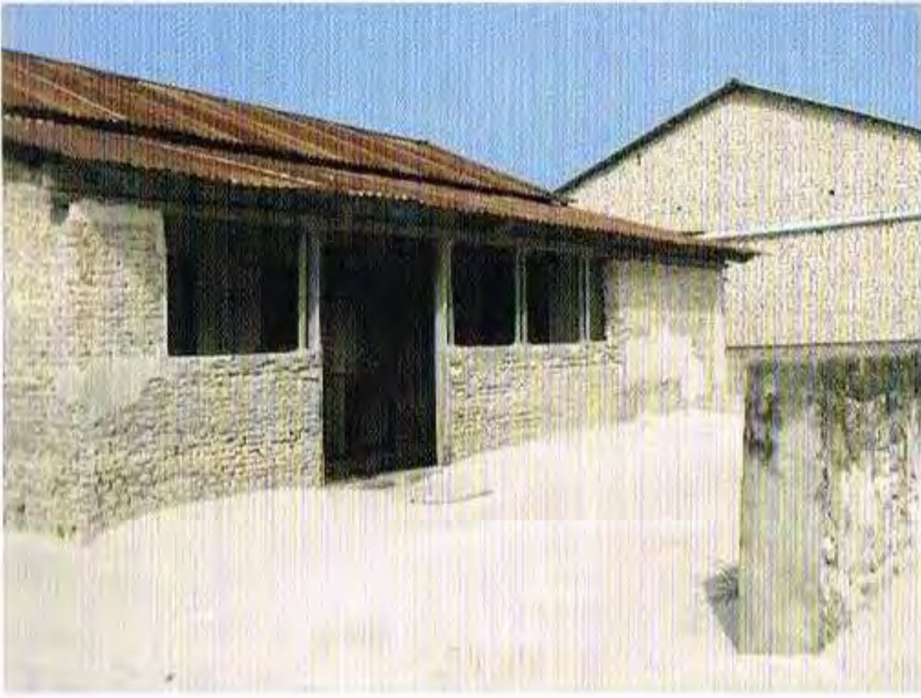
Image 6: Chipped coral masonry construction
